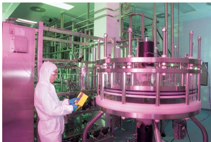
Fig. 1: A 1.2m diameter chromatography column used in large scale purification of a biopharmaceutical protein illustrating the approach to scale up of increasing column diameter to achieve larger column volumes.
